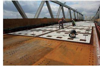
*Photo 2 : Precast slabs placed on the deck (photo : G. Forquet, Sétra)*
