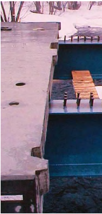
Fig. 2 Swedish prefabricated deck elements with dry joints.
