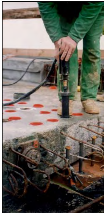
Fig. 3 French bridge where the studs are welded through holes after the elements are erected
