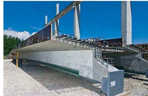
Fig. 5 Prefabricated VFT-girder, Germany. [2]
