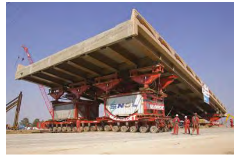
Fig. 4 Complete bridge prefabrication of 4500 South Bridge, Utah, USA. [1]
