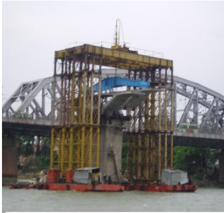
Fig 1: Erection of precast segment shell
